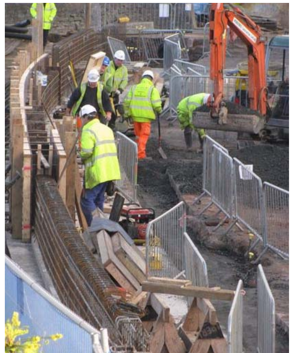
The base of the flood wall being constructed outside the Plough.
