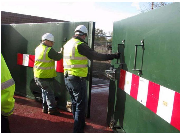
The New Street flood gate being closed
