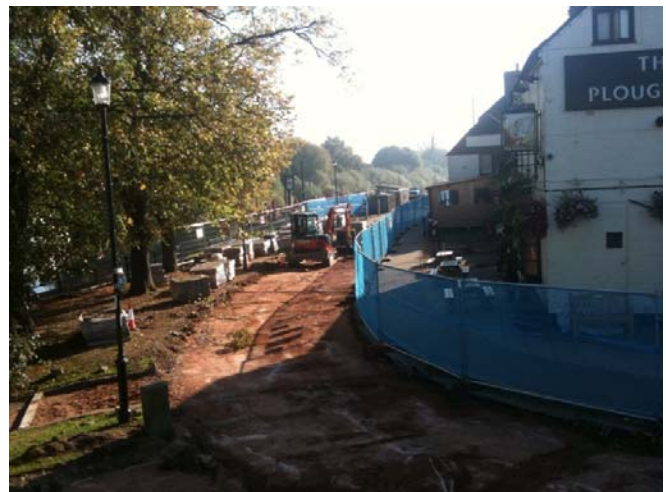
Site clearance works outside The Plough.
