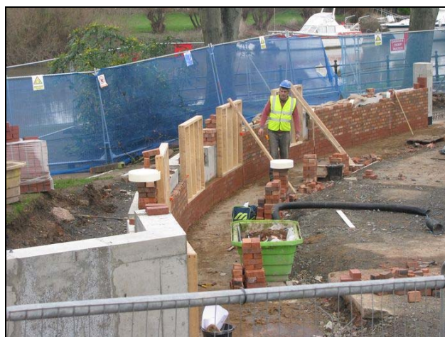
Photo 03: Brick cladding being added adjacent to The Plough.
