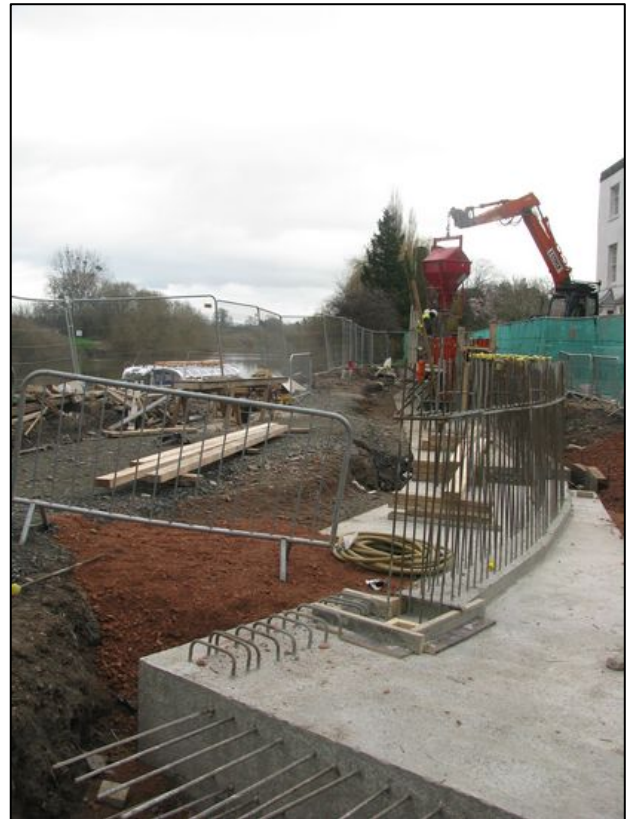
Photo 02: Progress adjacent to The Swan.
