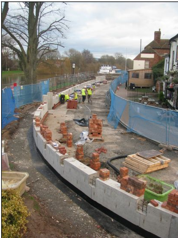
Photo 01: Work progressing outside The Plough.
